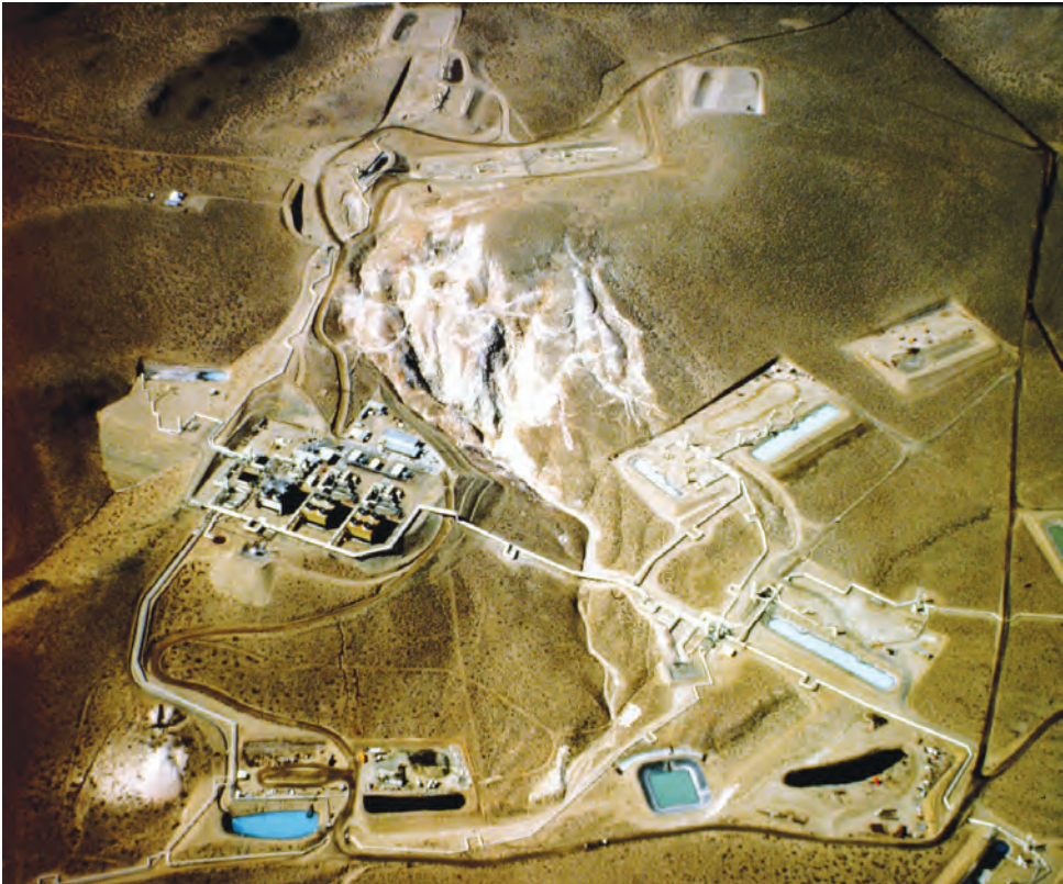
PHOTO: COURTESY COSO OPERATING COMPANY An aerial view of Coso Operating Company power plant “Navy 1,” one of four power plants that produce 175 gross megawatts (MW) of power.
