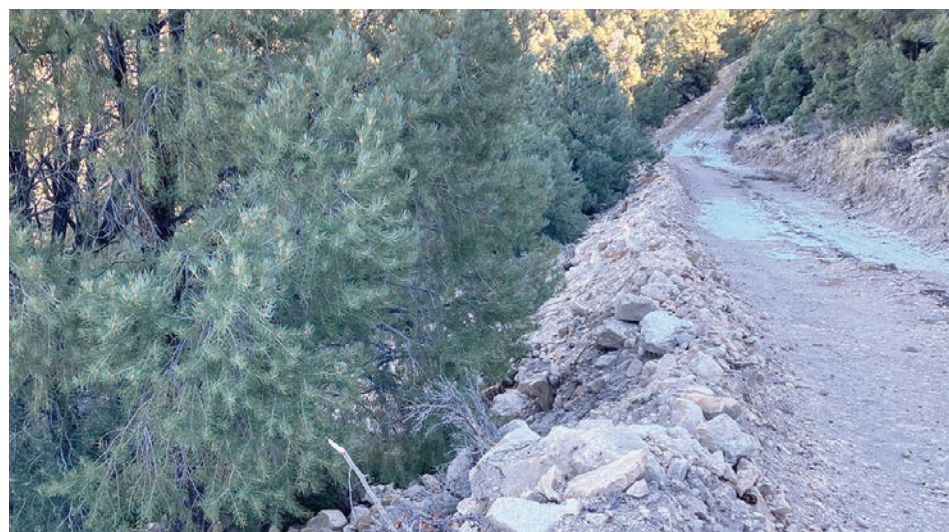
Road cut into steep hillside at Sawtooth Ridge
