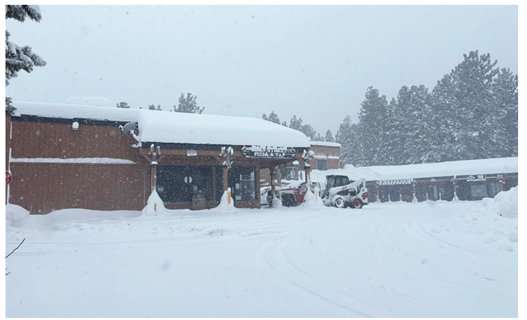
A blown transformer killed power on Main on Thursday had The Promenade looking empty and forlorn. Highway 395 between Mammoth and Bishop also closed Thursday.
