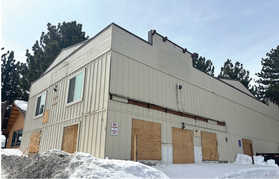
94 OMR next to and just below Nik ‘n Willies, the former site of a reservation company and the future site of Wind Drift Studios
