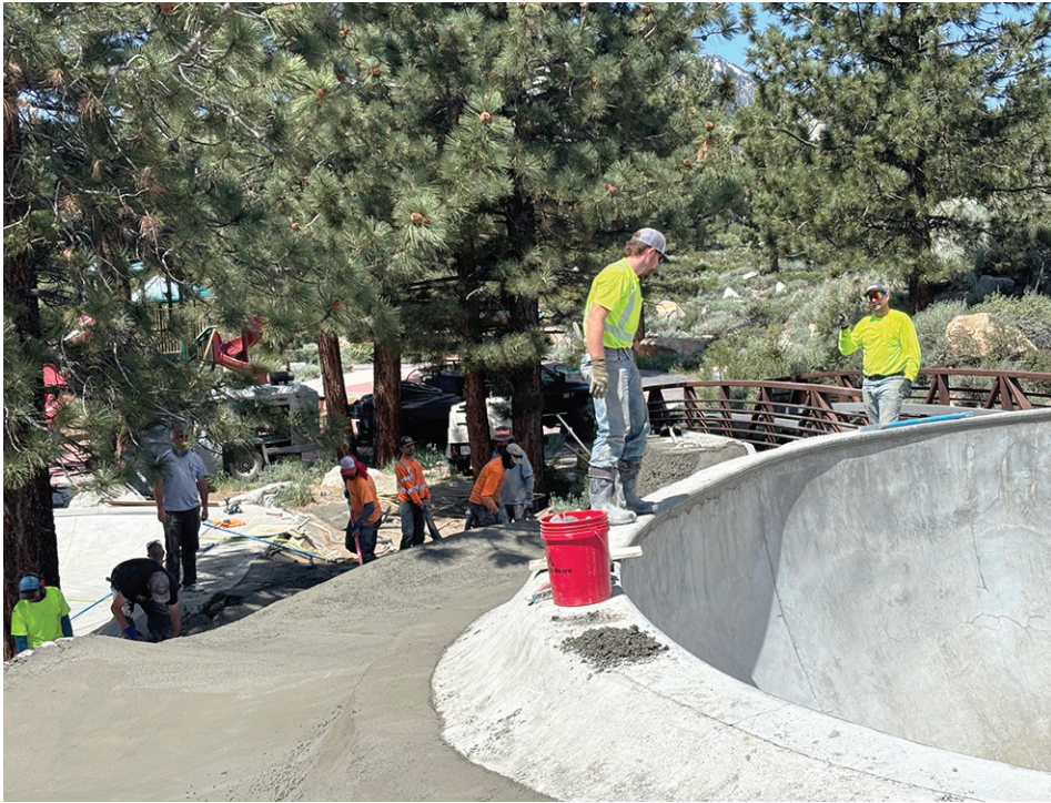
Crews have spent the past month or so working on a $75,000 overhaul of the Brothers Skatepark in Mammoth. During that time, the park has closed just one day, this past Monday.
