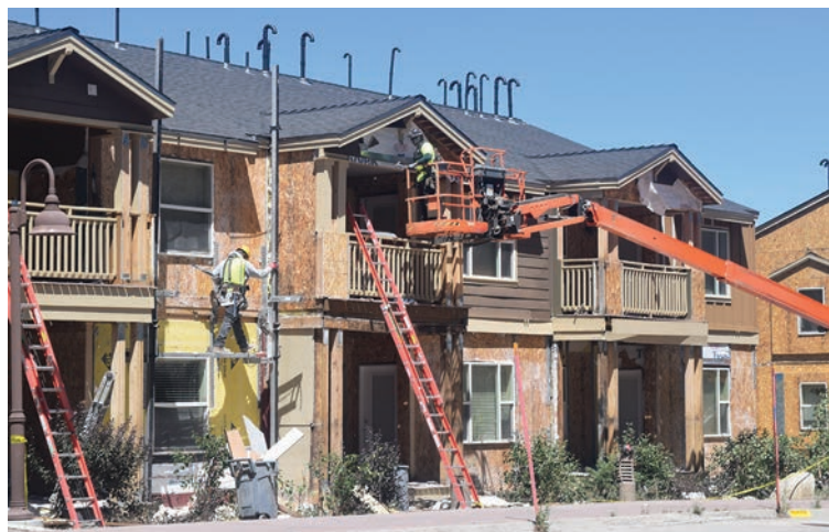
Construction crews strip the siding from the Aspen Village Apartments
