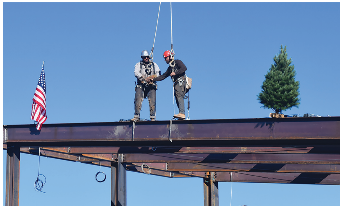
Construction workers shake hands as the final beam on the Southern Mono Hospital District North Wing project is placed on Friday afternoon, adorned with a tree and a flag per Scandinavian tradition.
