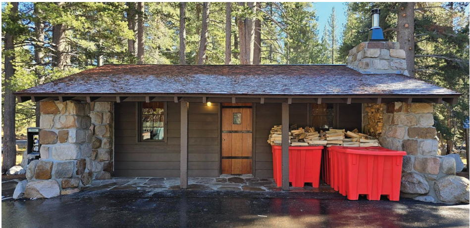
The Tuolumne Meadows Ski Hut post-renovation
