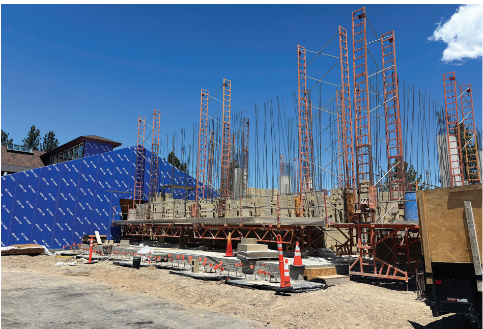
The MACC, currently under construction
